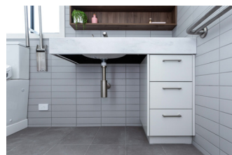
Accessible vanity with integrated basin.
