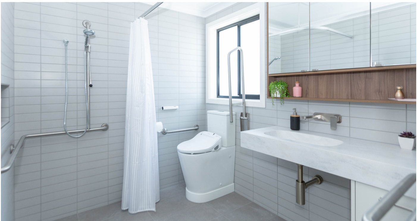
A fully accessible bathroom featuring hobless shower base with tile insert to point drain, toilet handrail, shower grab rail with hand shower, shower curtain and tiled shower storage niche.
